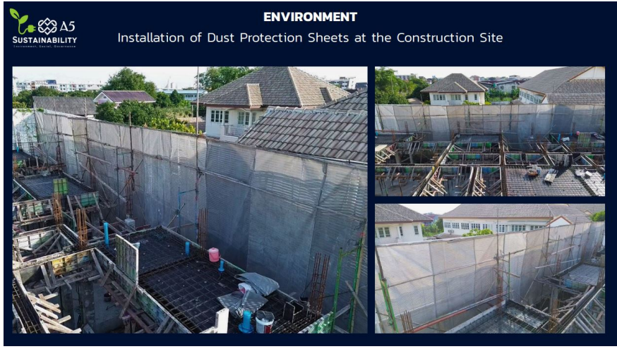
Installation of Dust Protection Sheets at the Construction Site
