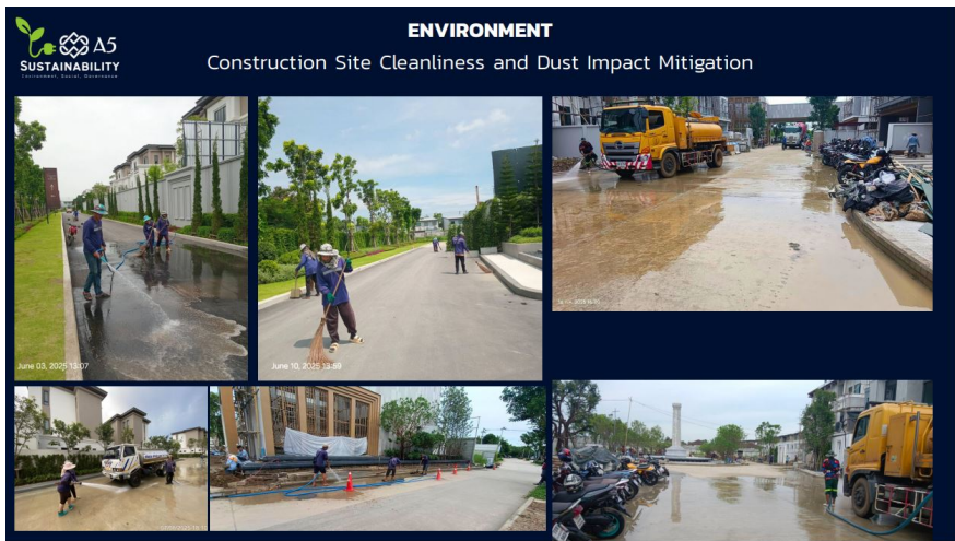
Construction Site Cleanliness and Dust Impact Mitigation
